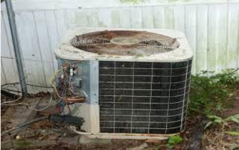
10 SEER Backup Heat @32F
