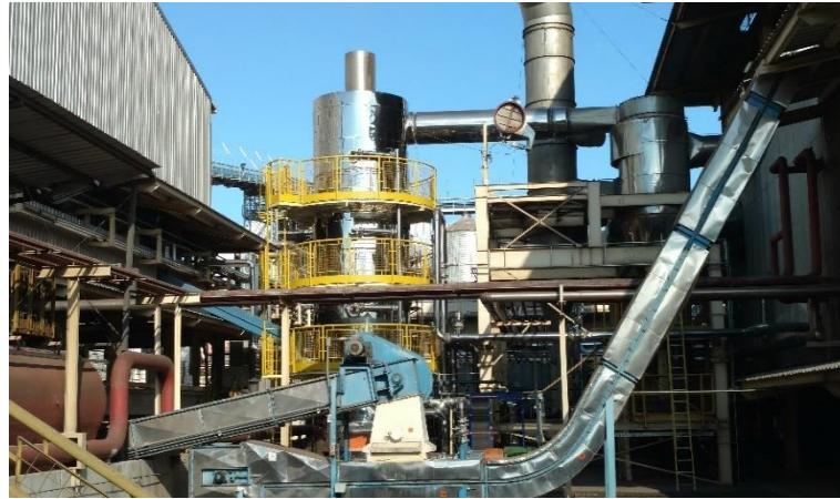
Dryer-Cooler Exhaust from DTDC in Soybean Oil Extraction
