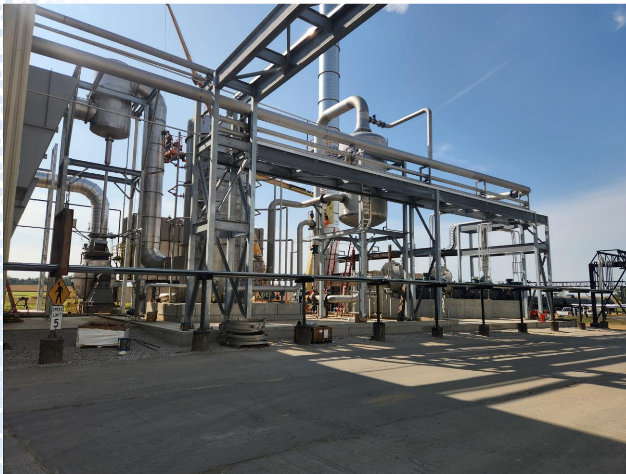
Steam-Generating Heat Pump under construction ("WHIR" System)
